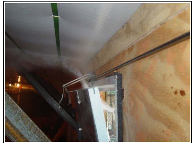
Figure 5. Air entering a house moving parallel to the side wall.
