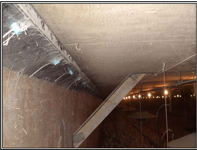
Figure 7. Continuous inlets tend to produce very small air jets which do not throw very far.
