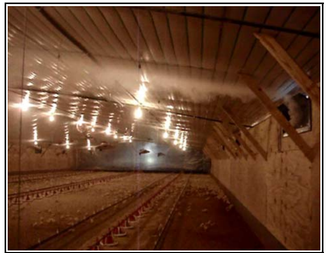
Figure 2. Optimal inlet air flow pattern during cold weather.
