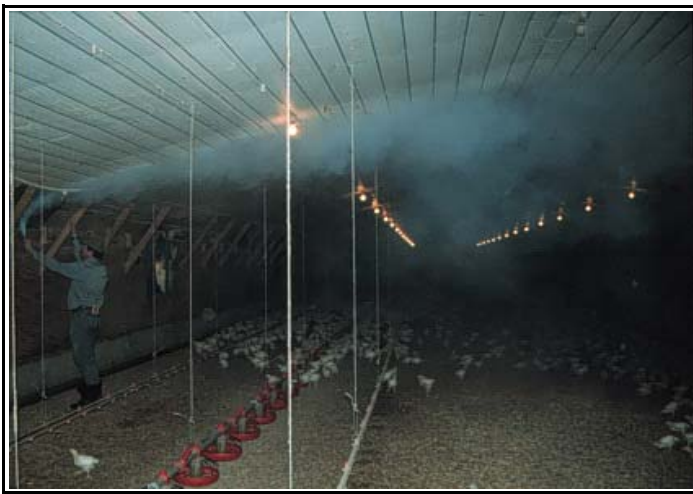
Figure 2. Optimal inlet air flow pattern during cold weather.
