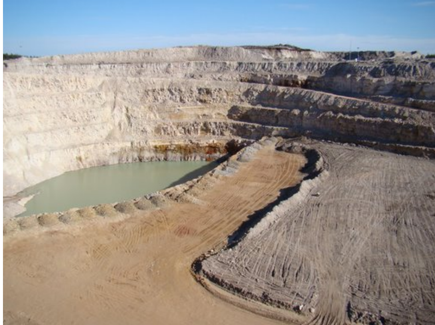
Fig. 6. Waste rock disposal at mined-out open pit at McClean Lake. Potentially acid-generating rocks are disposed of under water while non-acid-generating materials with low radioactivity are placed dry under a till cover.
