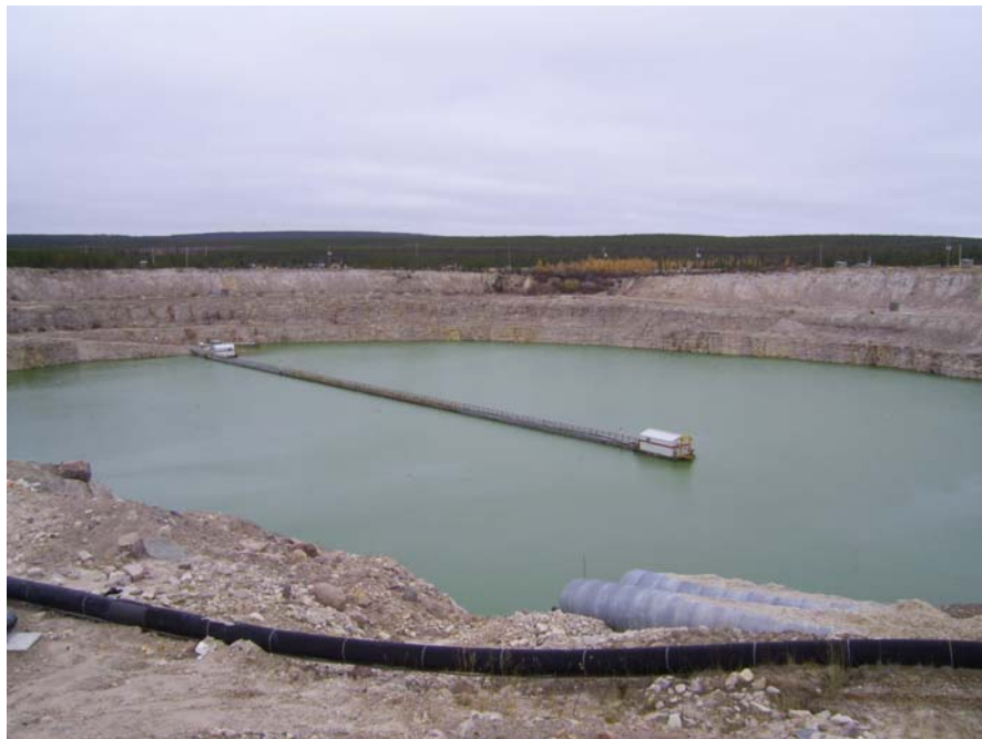
Fig. 7. In-pit tailings management facility (TMF) at McClean Lake. Water is pumped and circulated to ensure tailings consolidation at the pit bottom and designed water level is maintained in the pit lake.
