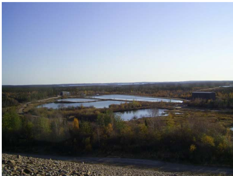
Fig. 8. Collection and polishing ponds at the Rabbit Lake Operation, Saskatchewan. Only water meeting applicable regulatory guidelines is discharged to the receiving environment.
