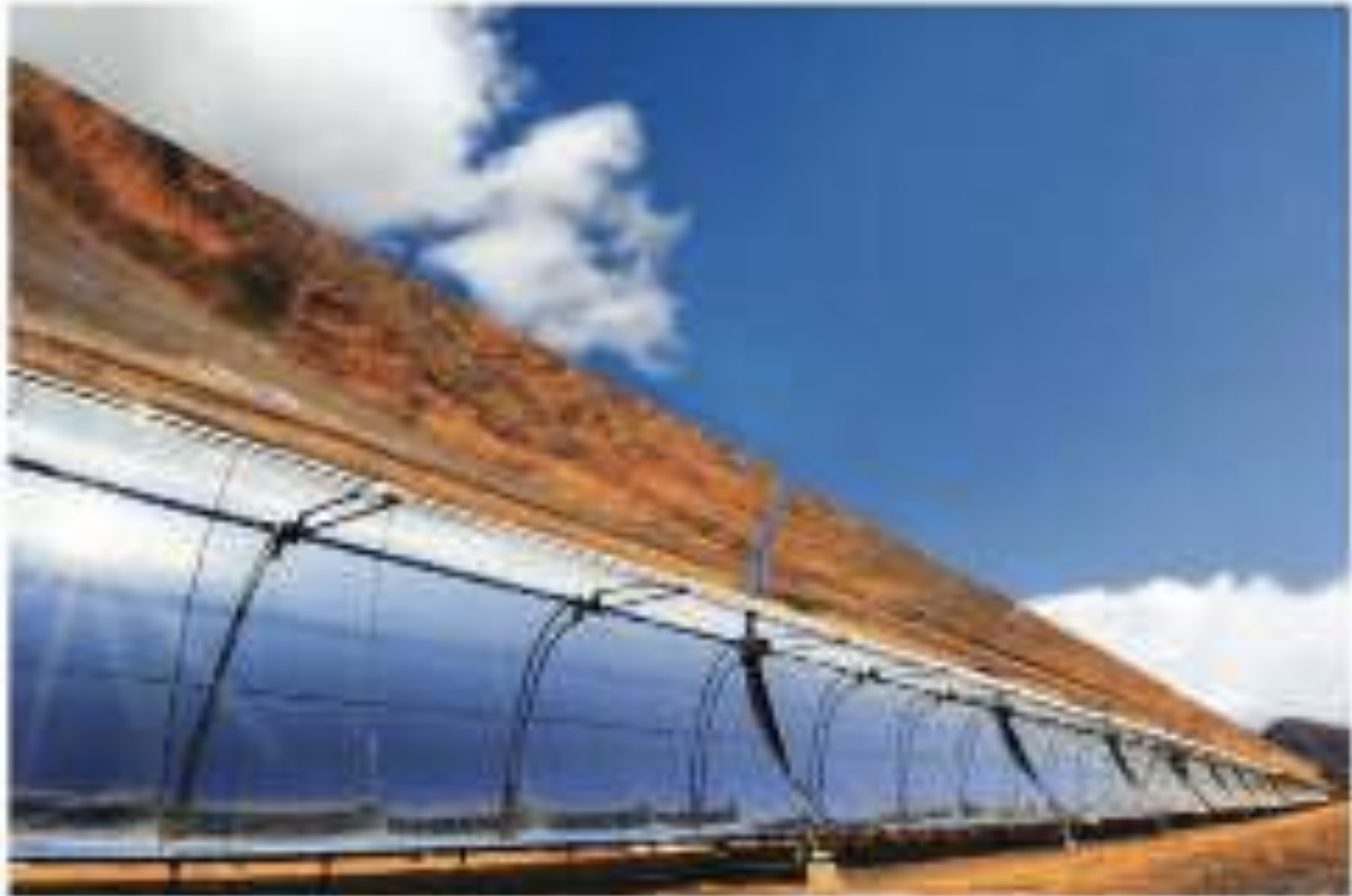
Figure 3.5 Solar receiver for trough technology (DLR, Markus Steur).
