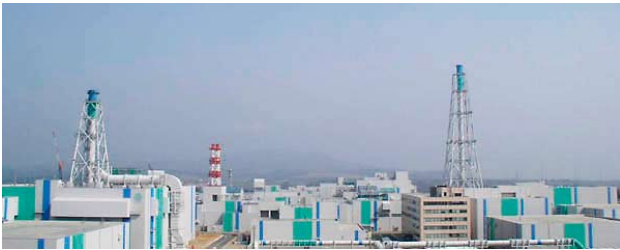
Fig. 3—Rokkasho Reprocessing Plant. A view of the Rokkasho Reprocessing Plant (source: Japan Nuclear Fuel Ltd. web site). The facility has a maximum annual capacity of 800 t of uranium and incorporates technologies from France, the UK, Germany, and Japan.
