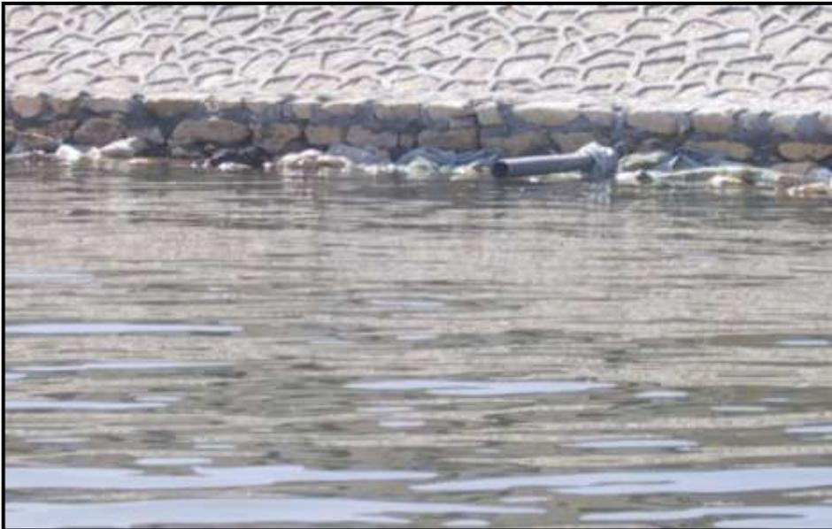
Photo (1). Sewage Network Outfalls in Rosetta Branch
