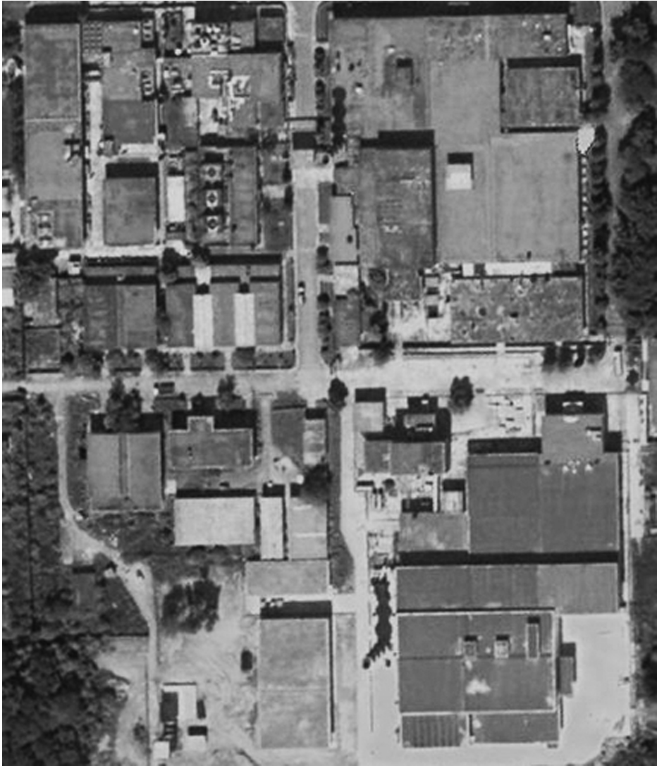
Figure 3: Original reprocessing plant (top right) and possible new reprocessing plant (bottom right) at the New Labs site, Rawalpindi, September 2006 (Google Earth imagery, courtesy of ISIS).
