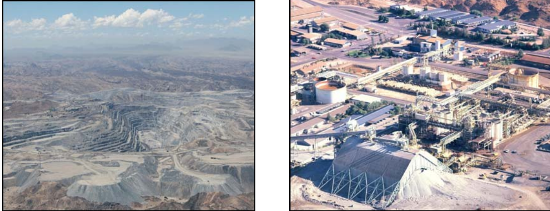
Plate 4.3: Aerial views of Rössing mine and part of the Rössing plant. Much of the total footprint of 24 km 2 is taken up by waste rock dumps (photo SAIEA and Rössing).
