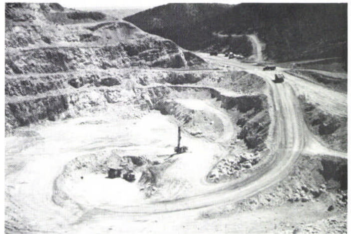
FIGURE 2. The open-pit Ortiz mine of Gold Fields Operating Co.—Ortiz, Old Placers district (#6, Fig. 1). Gold Fields mines about 3,000 tons of ore a day running about 0.05 oz/ton (1.8 ppm), making this the tenth largest gold producing mine in the U.S. in 1982. Photo by Susan Beattie. Published with permission and through the courtesy of Gold Fields Operating Co.—Ortiz.
