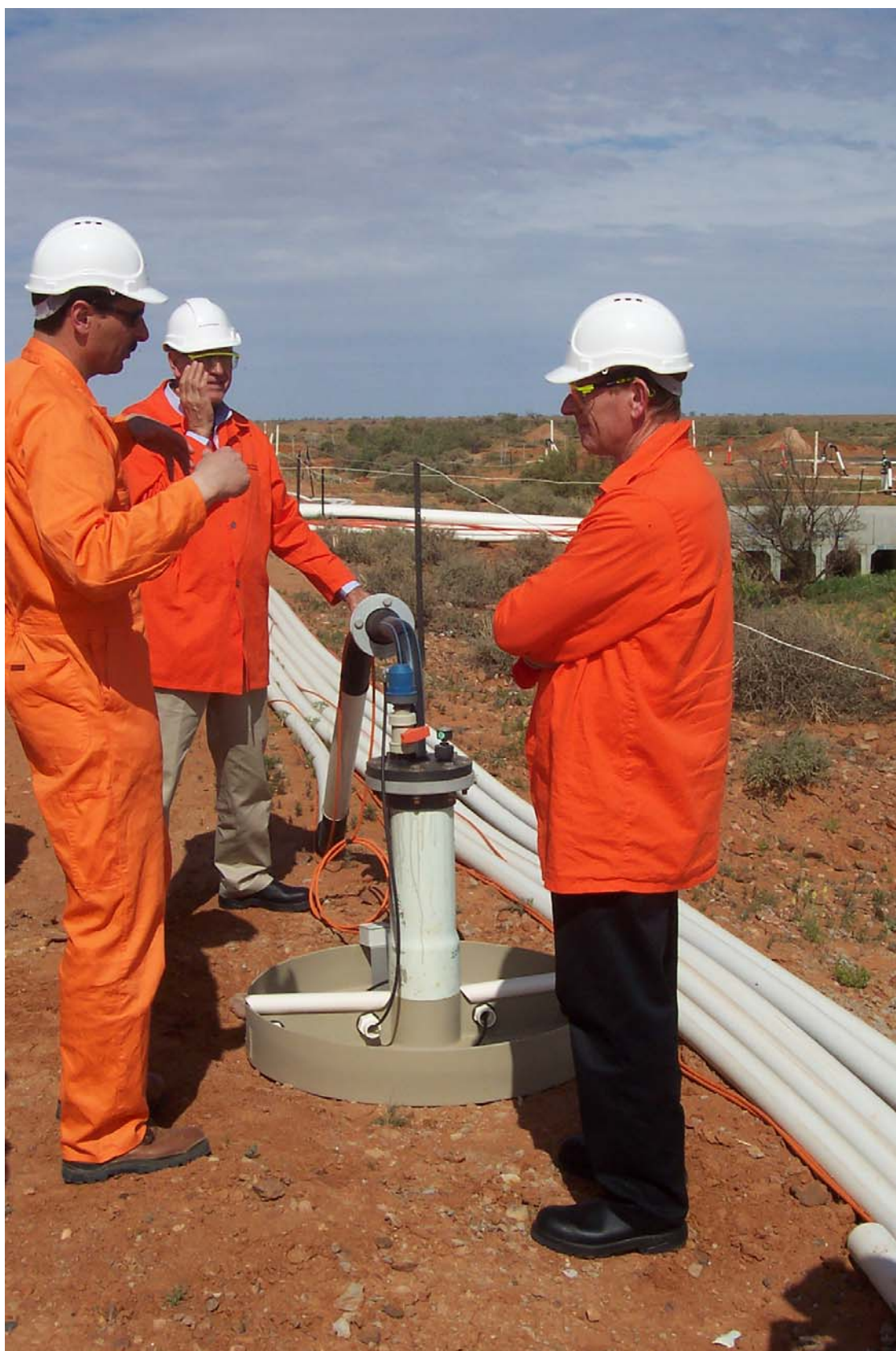
Figure 3.9 Committee members inspecting an extraction well at the Beverley in-situ leach uranium mine in South Australia
