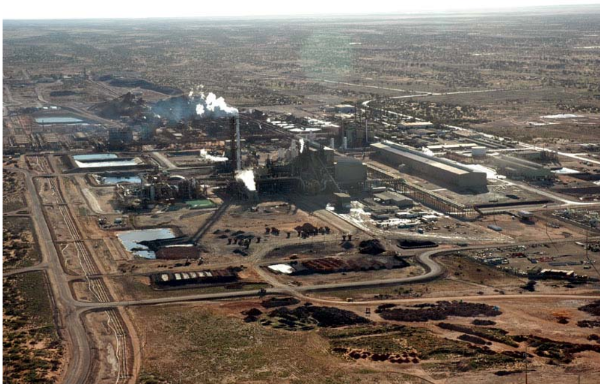
Figure 3.8 Aerial view of Olympic Dam
