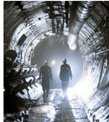
Mining tunnel in Cigar Lake
