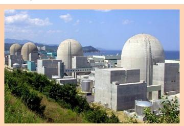
Power : 1,000 MWe Life Time : 40 years Const. : 51 months Seismic : 0.2g (5.6)\* APR1400
